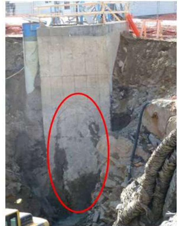
**Photograph of concussive blast damage to existing wet well.**
