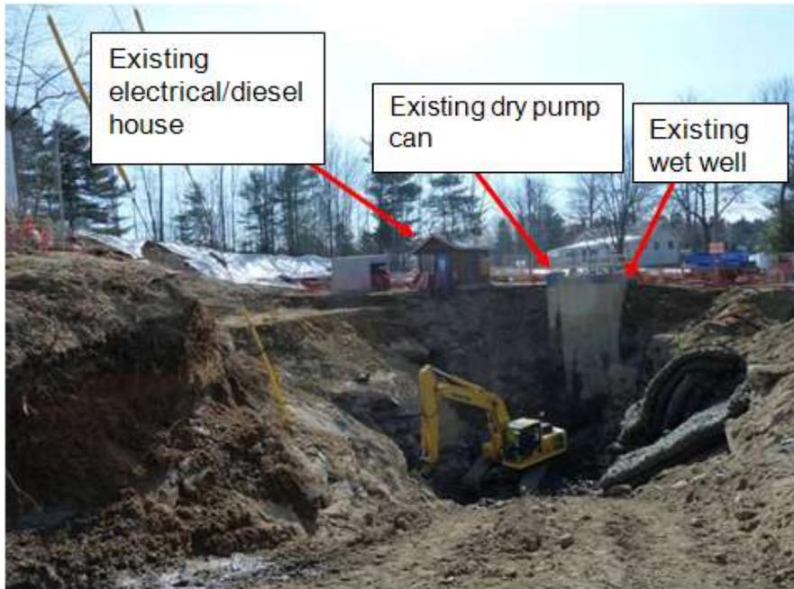
**Photograph of sewage pumping station site including pit where rock blasters was blasting, existing wet well, existing dry pump can and existing electrical/diesel house.**
